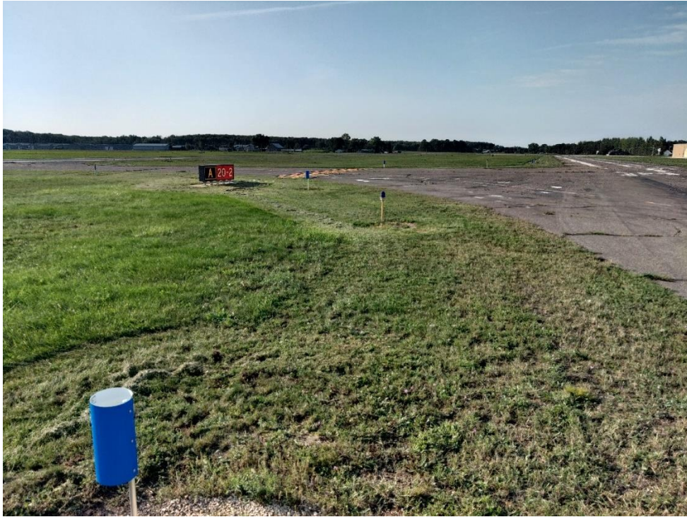
Photo 3: Overview, West of Central Runway, Facing North
