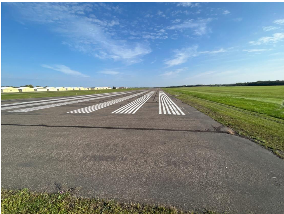
Photo 4: View of Runway from Southern End, Facing North
